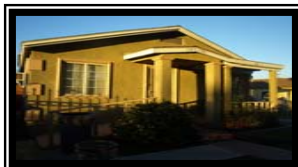
Premier Transitional Care House
